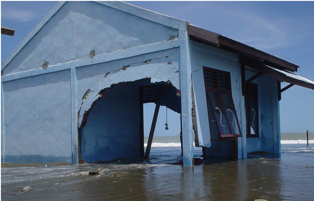
Figure 5.2 New buildings destroyed by flooding in 2007 in Meulaboh. Source: author.
