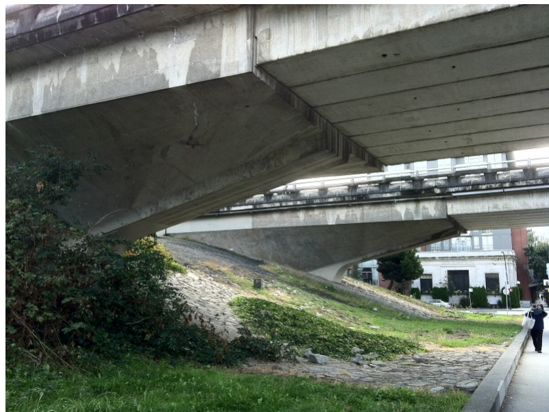
Figure 1.4 The Georgia and Dunsmuir Viaducts
